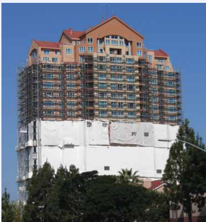
The remediation of this condo offered several challenges, including construction of an exterior containment system upon 21 story scaffolding.
