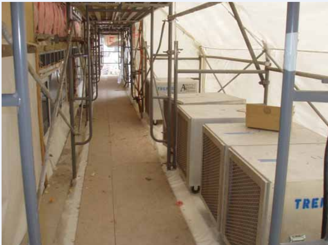
To save the cost of relocating residents, the remediation crew created a negative-pressurized containment around the exterior of this condo.
