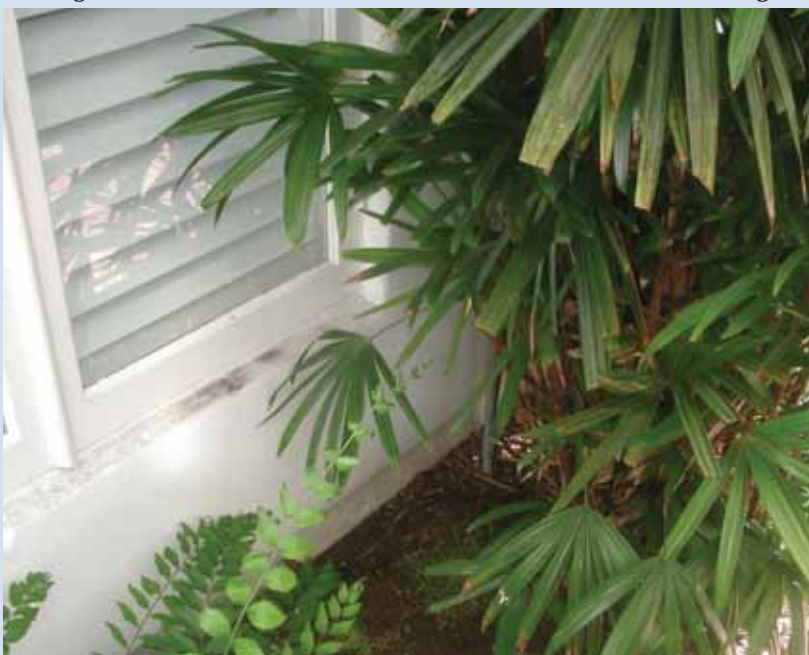
Lush vegetation hid the beginnings of wood rot on this French door.
